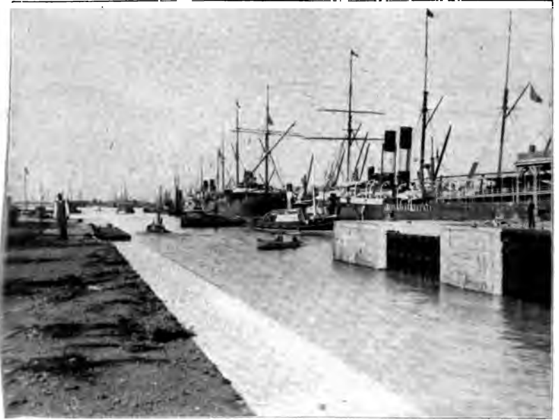
ENTRANCE TO DOCK No. 1 (BUENOS AIRES)
