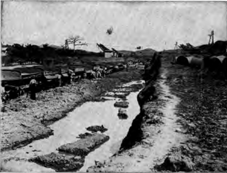
EXCAVATING FOR THE PANAMA CANAL
