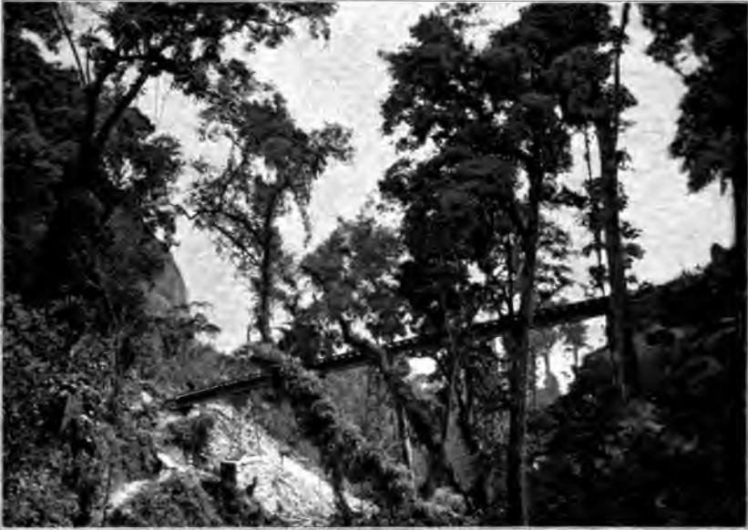
RAILWAY VIADUCT NEAR PETROPOLIS—"WE GO OVER RAVINES"
